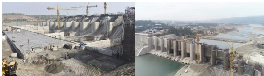
Fig. 8. Construction work of dam project
