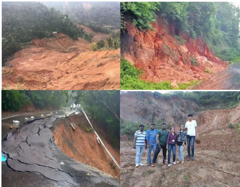
Figure.4. Photographs of Landslides
