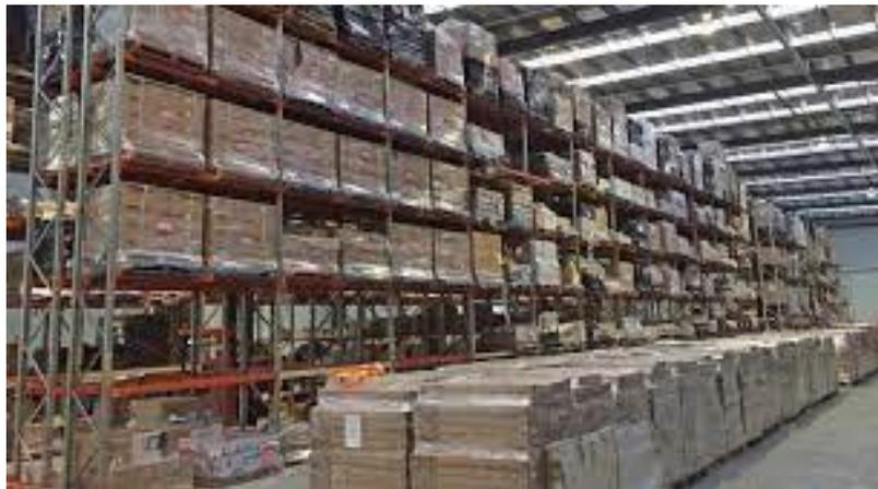
**Fig. 4.** Overloaded warehouse, present loading condition may be beyond the design load
