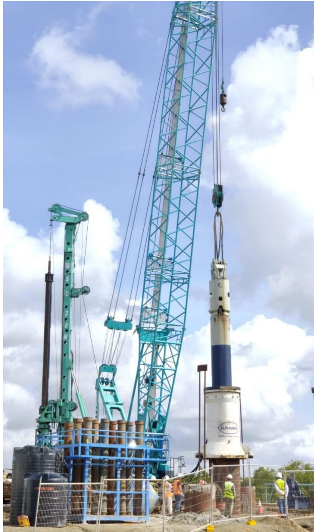
Fig.2. Typical set up for Dynamic test
