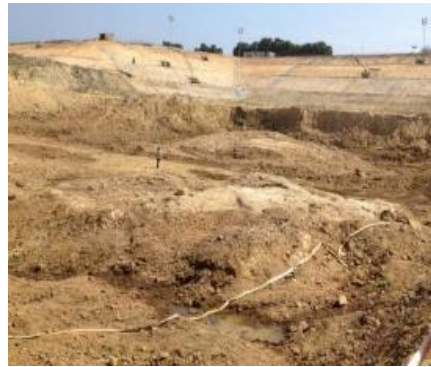
Fig. 1. View of the excavated pit
