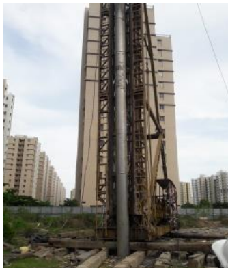
Fig. 1: Pile casing driving at Newtown, Kolkata by Impact Hammer
