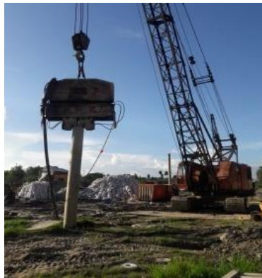
Fig. 2: Pile casing driving at Baruipur, South 24 Parganas by Hydraulic Vibratory Hammer
