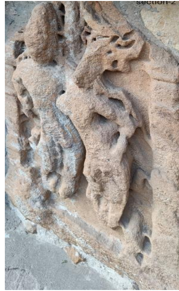
Fig. 10 Slight deterioration in the carvings
