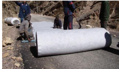
Fig. 6. Geocomposite Drain being rolled out for cutting
