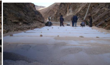
Fig.7. GCD laid in slope and being covered by sand layer
