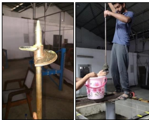
Fig. 3. Excavation of saturated soil using auger boring
