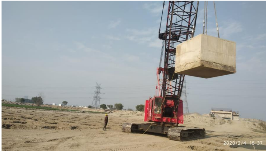
Fig. 6. Dynamic compaction at the site in progress
