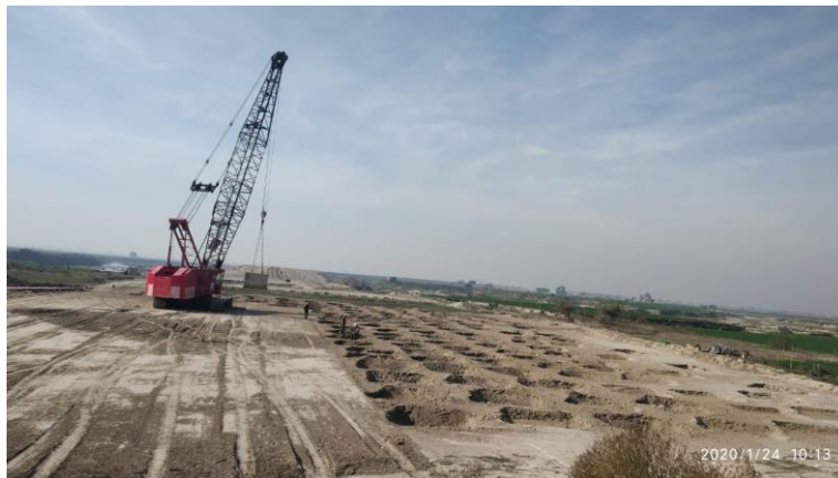
Fig. 5. Dynamic compaction at the site in progress
