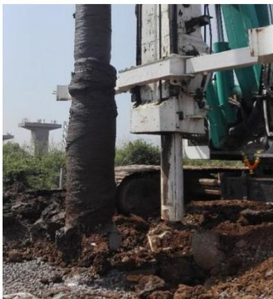
**Fig. 8.** Rotating Screw Assembly
