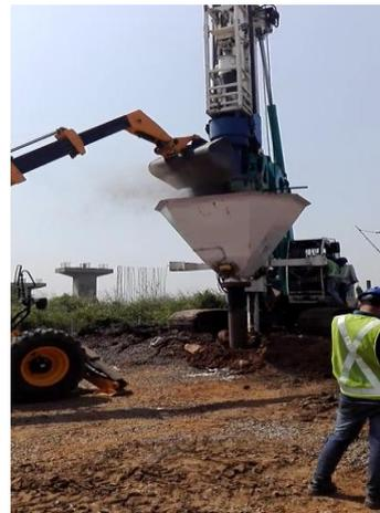
**Fig. 7.** Loading of Stone into the Hopper
