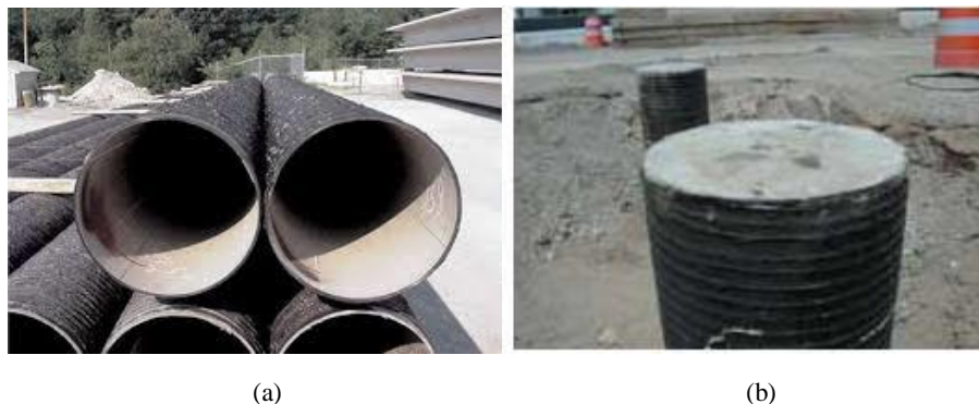
Fig. 2. FRP composite pile (a) Hollow FRP pipe, (b) Concrete filled FRP pile [14]
