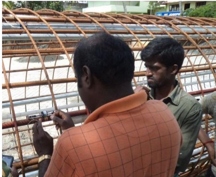
Fig. 1. Strain gage installation in progress
