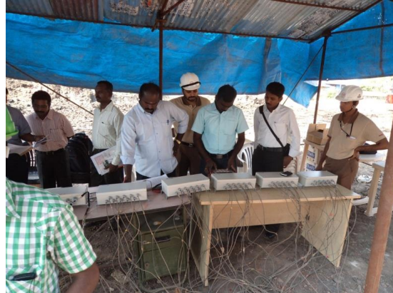
Fig. 3. Instrumented vertical load test – data collection in progress
