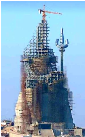
Fig. 11. Construction in progress
