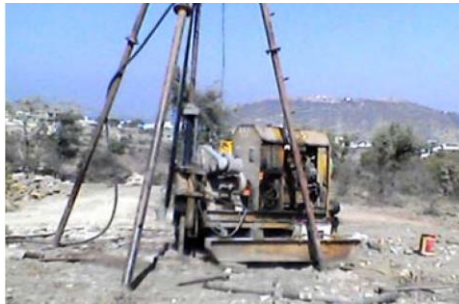
Fig. 5. Drilling in progress
