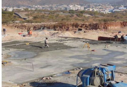
Fig. 8. Foundation level preparation
