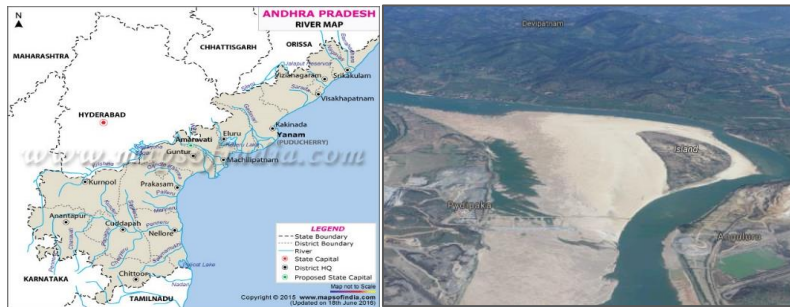
Fig. 1. Location of ECRF DAM at Polavaram
