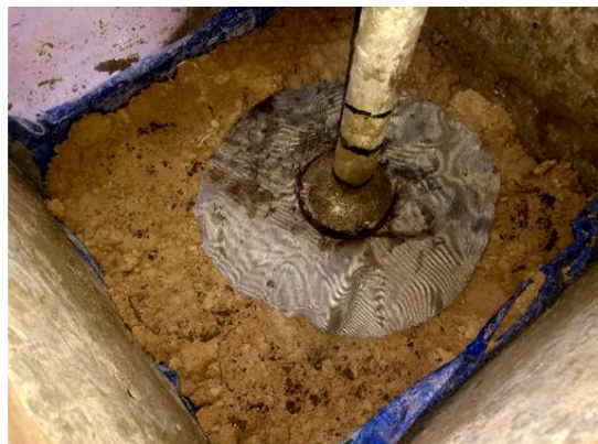
Fig. 3. Positioning of anchor before placing the soil mass
