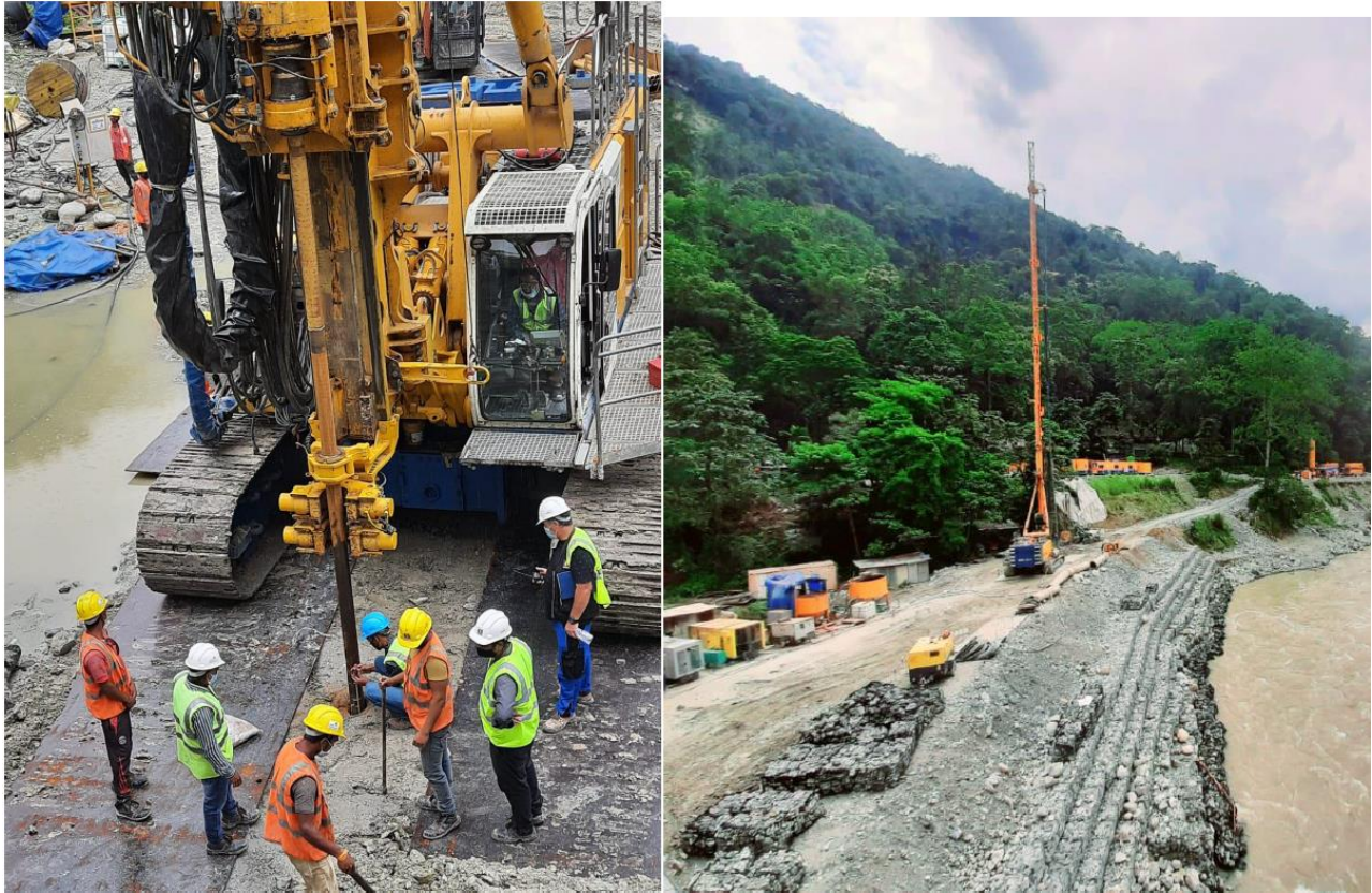
Fig. 10 Redrilling for Jet Grouting and Predrilling of the Holes in the Boulder Strata along the alignment
