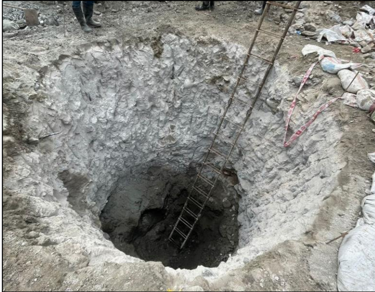
Fig. 4. Visual Inspection of Seepage
