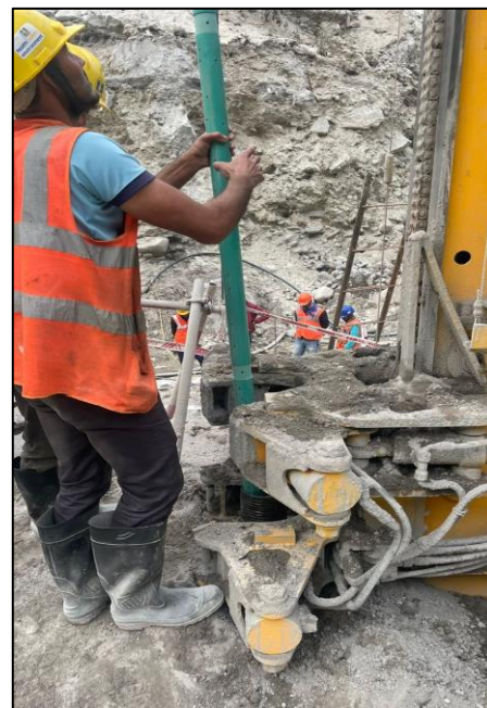
Fig 3b. Installation of perforated pipe
