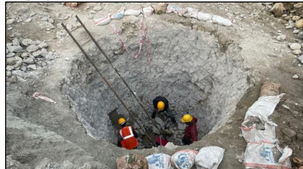
Fig. 2. Excavation of Shaft
