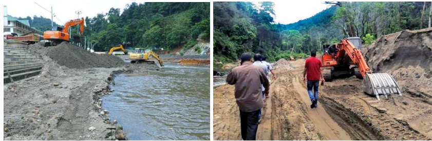
Fig. 1. Dredging of flood Sediments and Removal Activities at the Pampa- Triveni [1]
