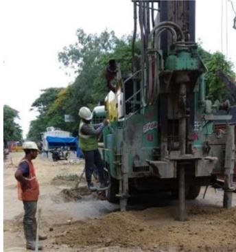
a) Rock anchor drilling in progress borehole
