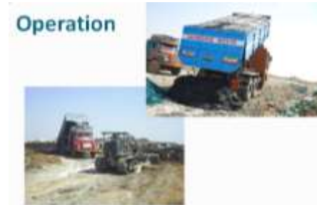
Fig. 11. Waste filling operation
