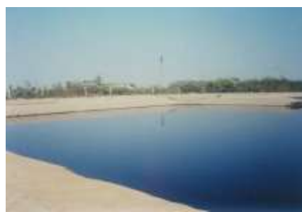
Fig. 18. Leachate solar pond
