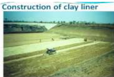
Fig. 8. Construction of clay liner
