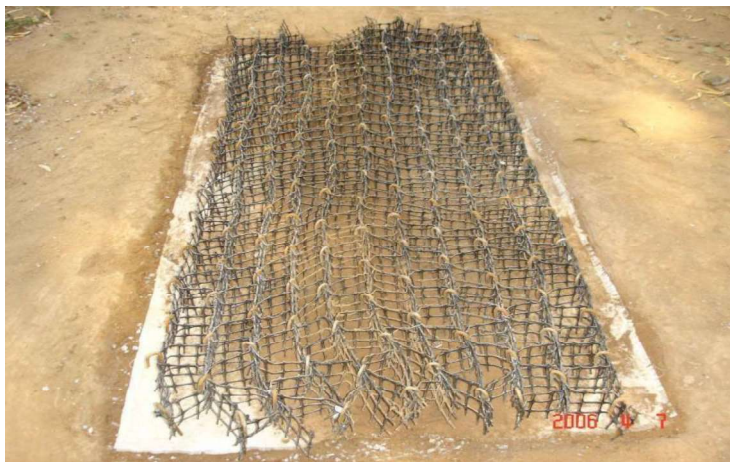
Fig. 11. Geocell layer prepared at the site
