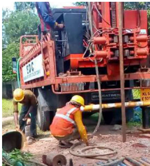
Fig. 9. Confirmatory soil investigation in progress.
