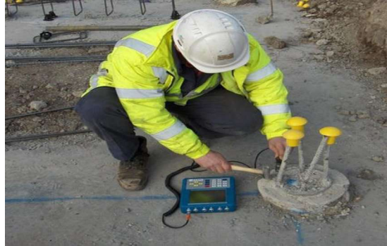
Fig. 8(a). Conducting pile integrity test on piles
