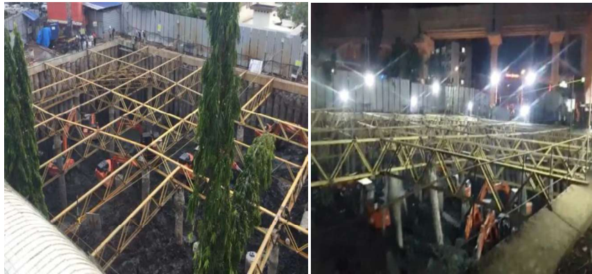
Fig 4. (a). Photos at different stages of touch pile system failure at Kaloor, Cochin
