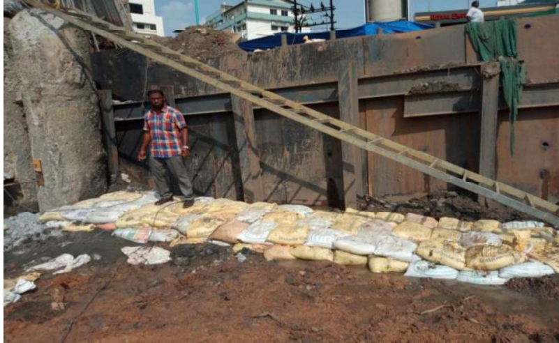
Fig. 6. Two-layer braced sheet pile system adopted near public road
