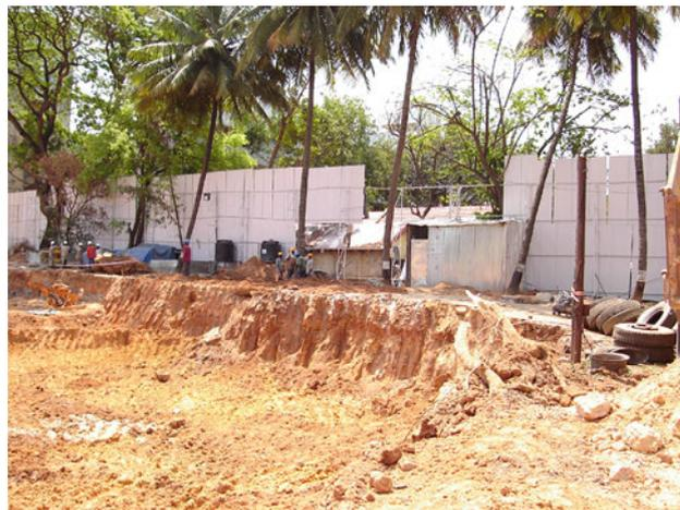
**Fig. 78** Excavation for grouted nails at Bangalore
