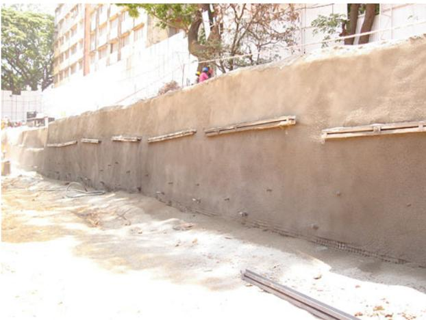
Fig. 80 Shotcreted surface after two rows of grouted nails
