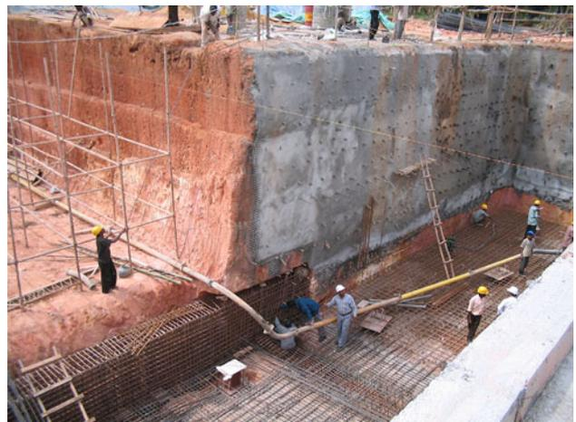
**Fig. 73** Protection of deep excavation at Air force station by driven nails
