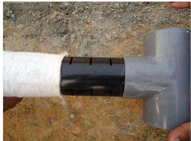
Fig. 48 Slotted pipes covered with geotextile
