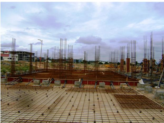
**Fig. 22** Reinforcement for raft
