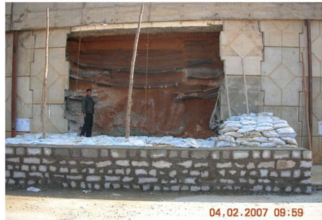
Fig. 12 Toe wall support at base for sand bags
