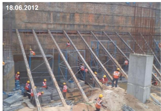
**Fig. 68** Removal of earth shoring and building of RCC wall with structural shoring in position
