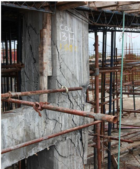
**Fig. 54** Crushing of the column due to uplift
