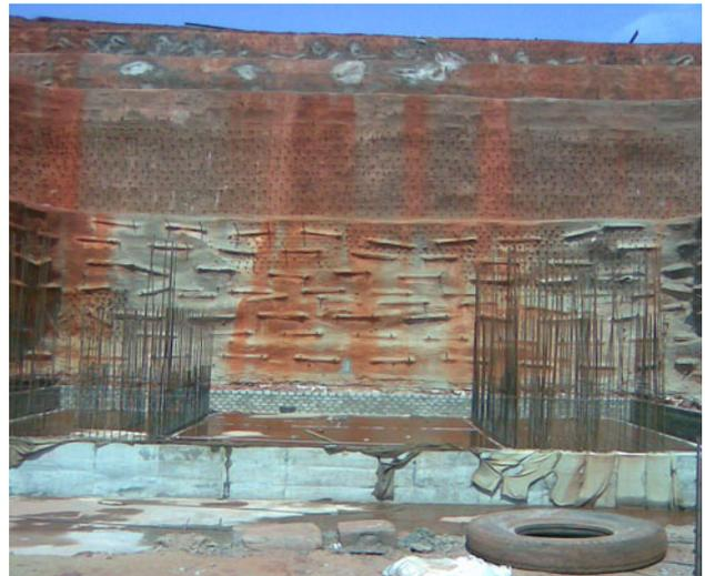
Fig. 82 Slope protection at NMDC project -Combination of driven and grouted nails
