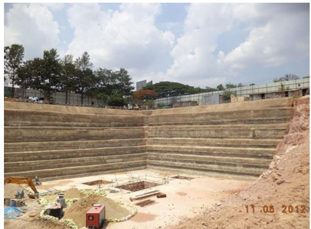
Fig. 83 Deep excavation with driven and grouted nails as finished
