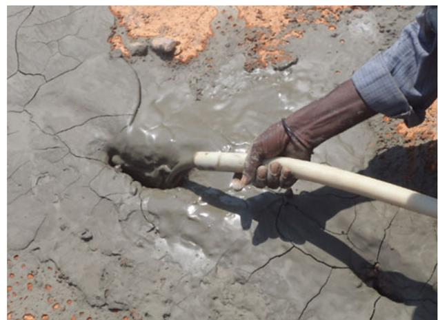
**Fig. 63** Grouting of the cracks
