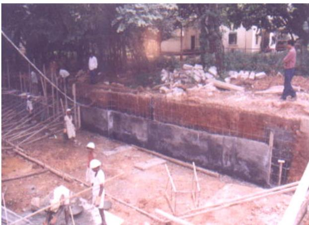
**Fig. 71** Concreting of the facing element at IISc
