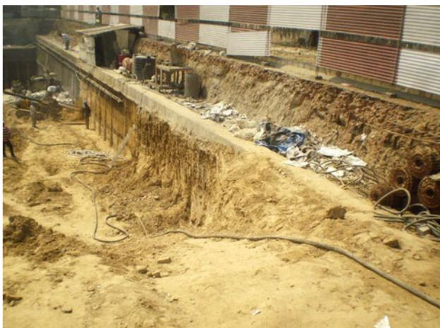
**Fig. 37** Installation of grouted nails
