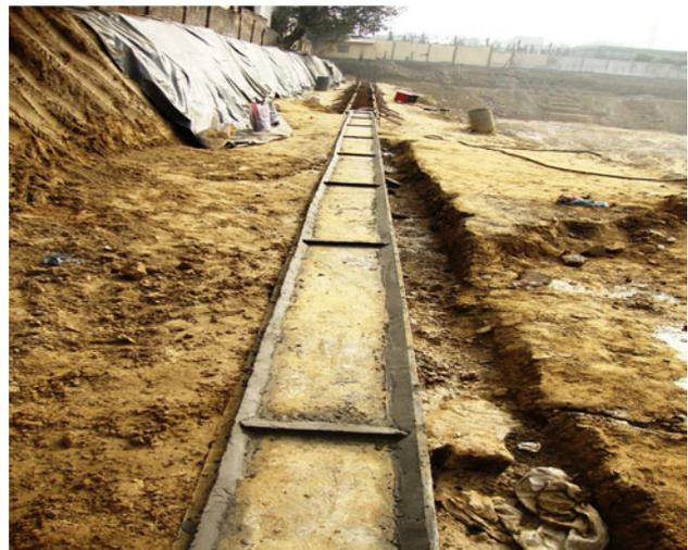
Fig. 35 Capping beam on piles
