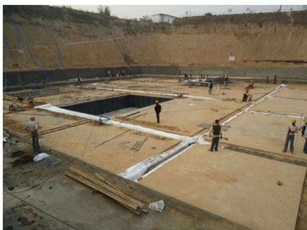
Fig. 47 View of the under slab drains
