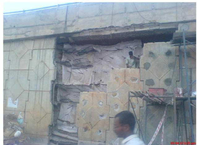
Fig. 17 View of replacement of facing elements
