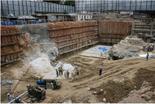
**Fig. 85** Touch piles of 300 mm size with grouted nails
