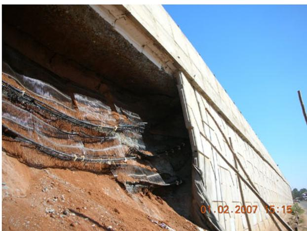
Fig. 8 Exposed friction slab
