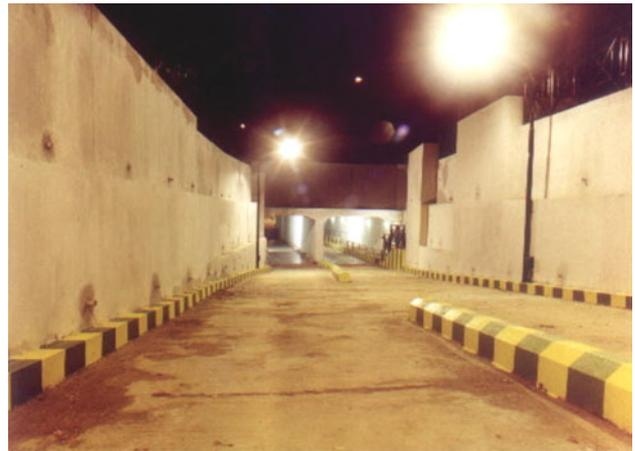
**Fig. 72** Finished ramp side walls for the underpass at IISc
