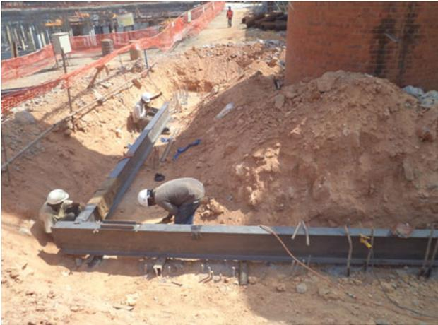
**Fig. 64** Capping beam on the RCC piles
