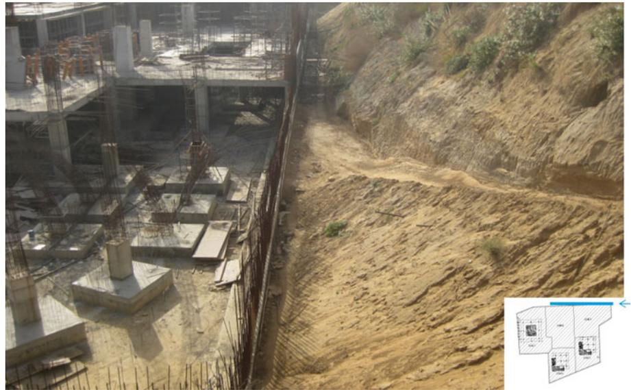
**Fig. 51** Backfill over garland pipe (another view)
