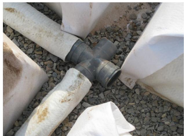
Fig. 49 Under slab drainage junction
