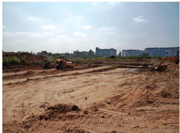
Fig. 19 The surface soil stripped to a depth of 2 m
