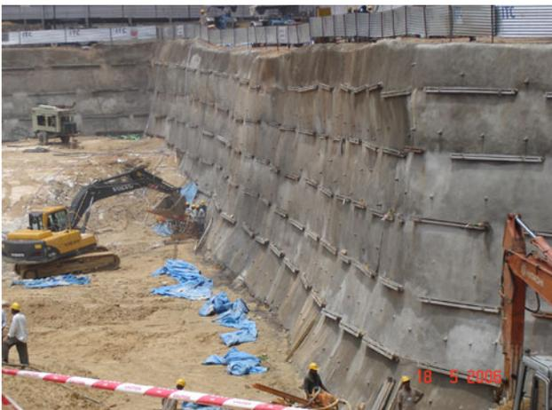
Fig. 81 Deep excavation and grouted nails as finished
