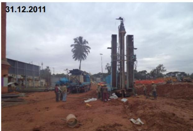
**Fig. 56** Installation of micro piles
