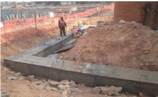
**Fig. 65** Capping beam on the RCC piles
