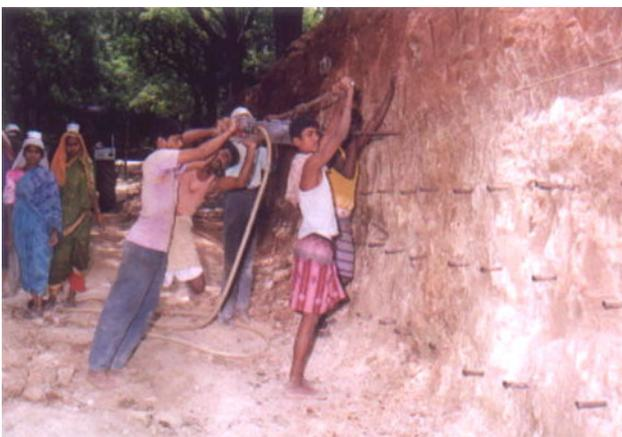
**Fig. 70** Driven nails for the ramp side walls at IISc
