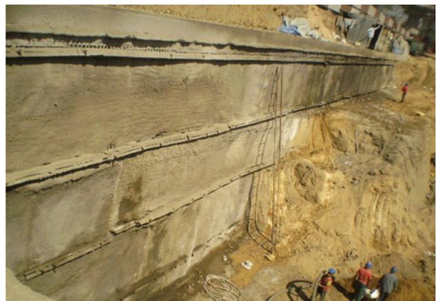
**Fig. 39** Installation of grouted nails with shotcrete in third row
