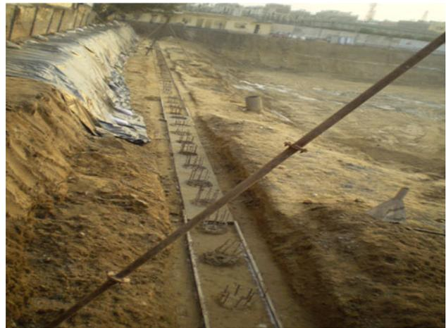
Fig. 34 Piles ready for capping beam
