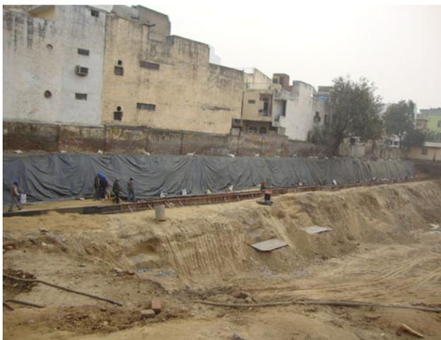
**Fig. 36** Building on the compound and excavation up to first benching
