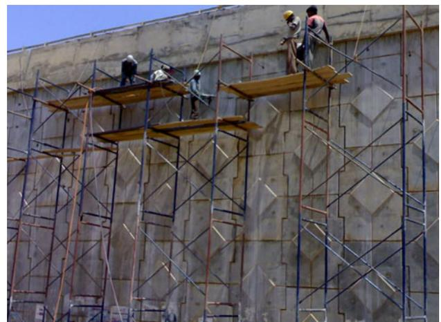
Fig. 18 Finished view of RE wall with additional driven nails
