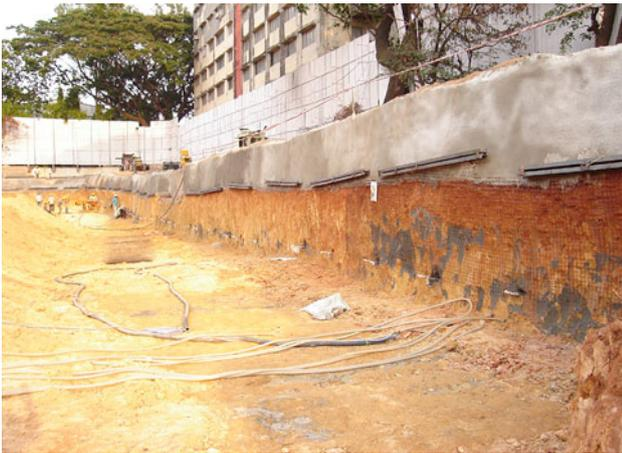
Fig. 79 Excavation and two rows of grouted nails
