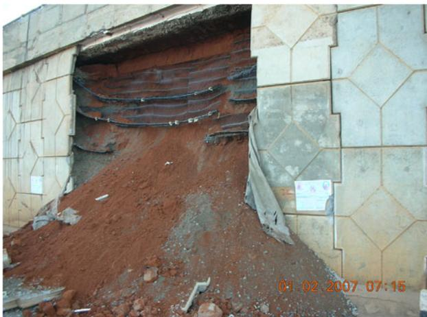
Fig. 7 Collapse of RE wall
