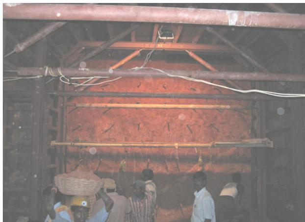
**Fig. 91** Driven nails to prevent collapse of excavation face
