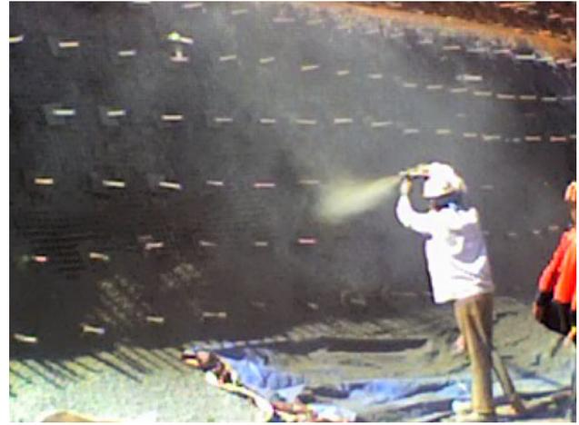
**Fig. 87** Slope protection at NMDC project
