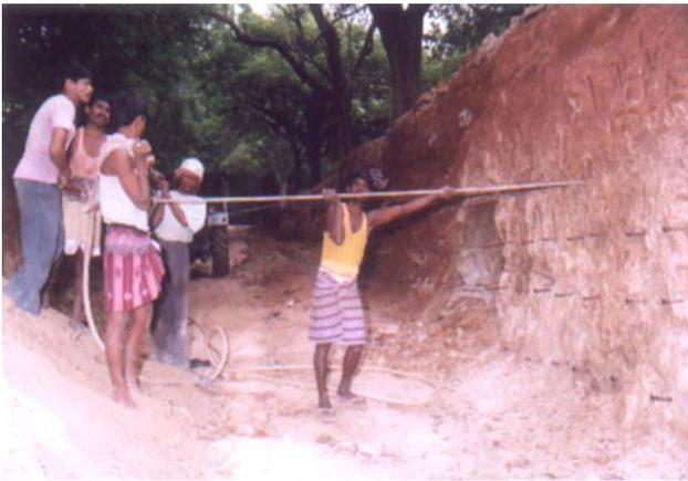
**Fig. 69** Driven nails for the ramp side walls at IISc
