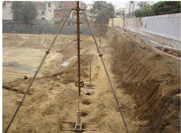
Fig. 33 Installation of piles
