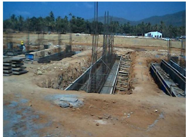
**Fig. 30** Construction of strip footing in the engineered fill
