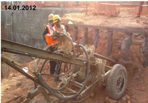
**Fig. 58** Installation of capping beam and first row of grouted nails
