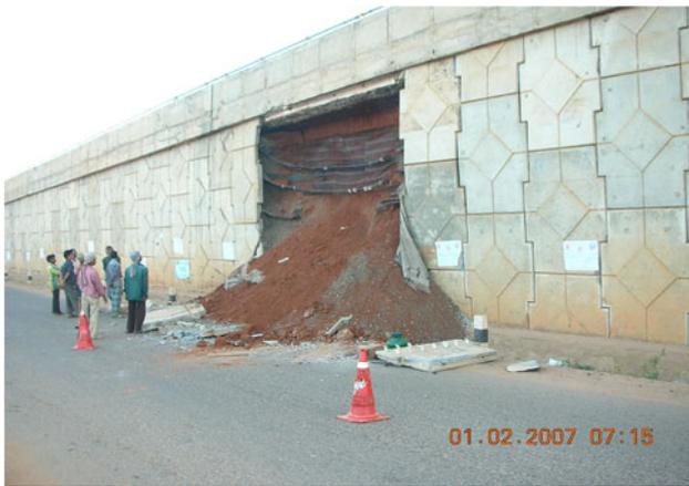
Fig. 6 Collapse of RE wall
