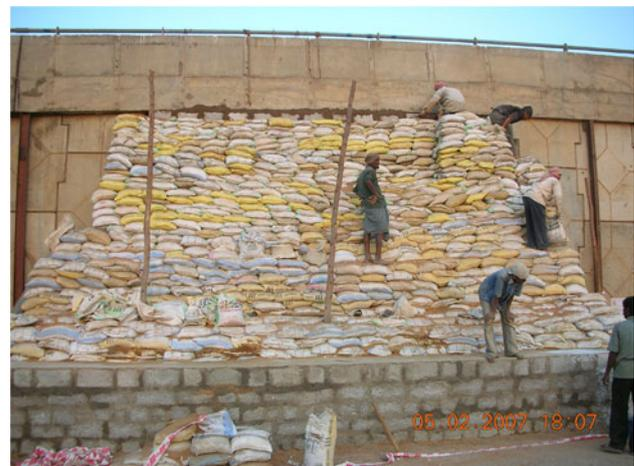
Fig. 13 Completion of sand bag shoring
