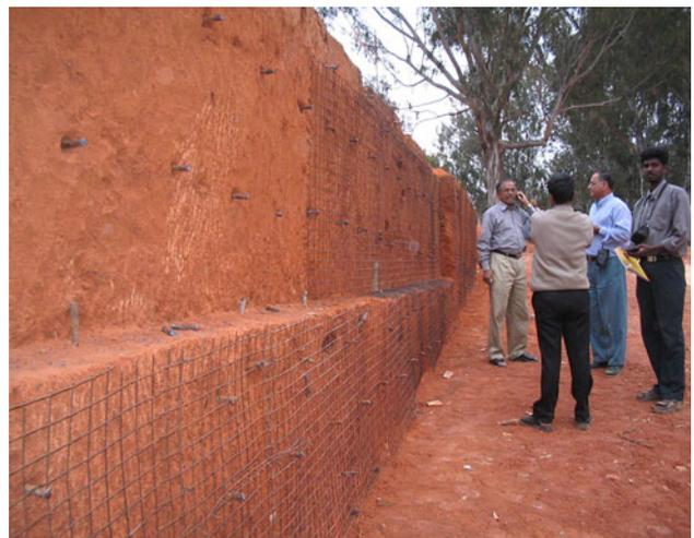
**Fig. 74** Protection of deep excavation at Air force station by driven nails
