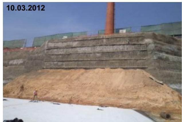
**Fig. 62** Earth shoring to control tilting of the chimney
