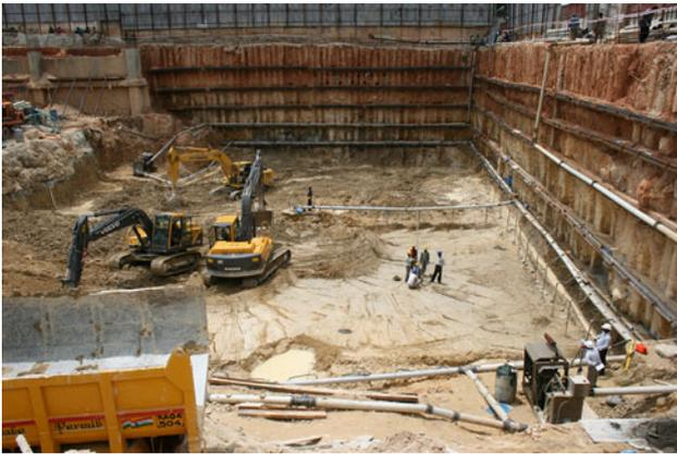
**Fig. 86** Touch piles of 300 mm size with grouted nails
