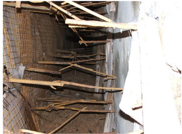
Fig. 16 Filling of sand in the gap behind the facing element
