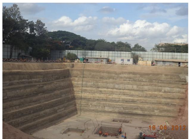
Fig. 84 Deep excavation with driven and grouted nails as finished
