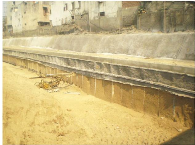
**Fig. 38** Installation of grouted nails with shotcrete
