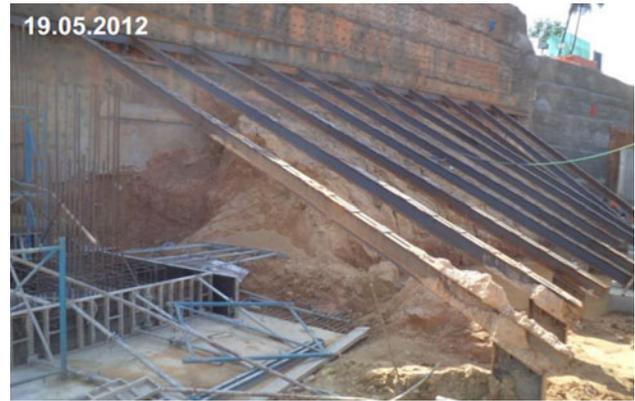
**Fig. 67** Removal of earth shoring and building of RCC wall with structural shoring in position
