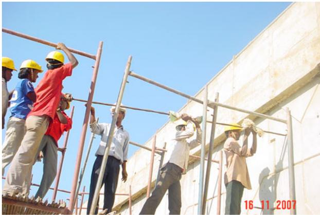
**Fig. 90** Driven nails to strengthen RE walls
