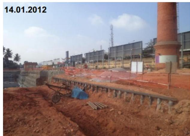
**Fig. 57** Installation of capping beam and first row of grouted nails
