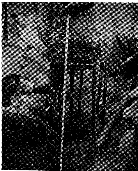
Figure 13. A cast-in-situ pile without toe concrete
