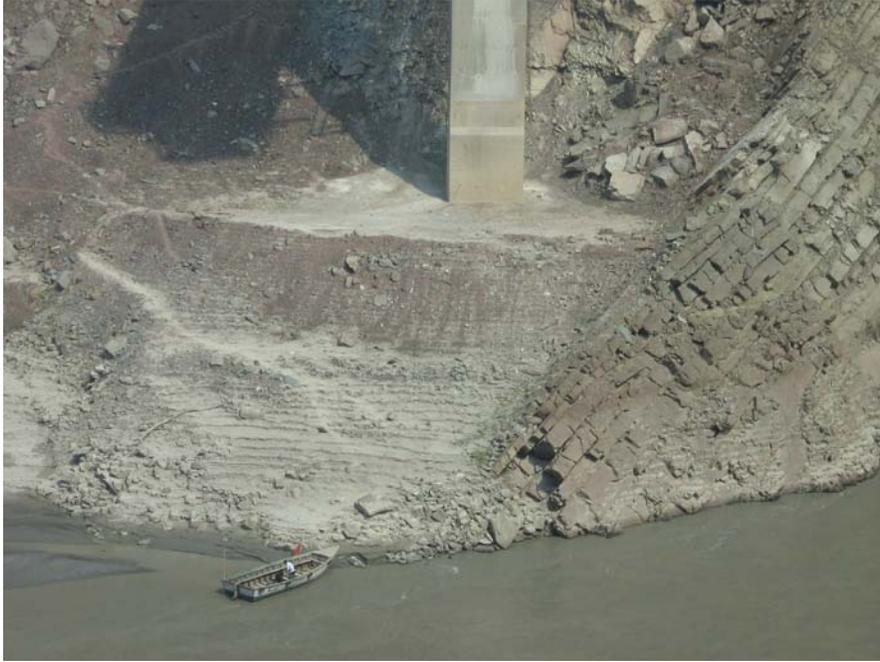
Fig.2. Heavily jointed rock mass below a bridge pier
