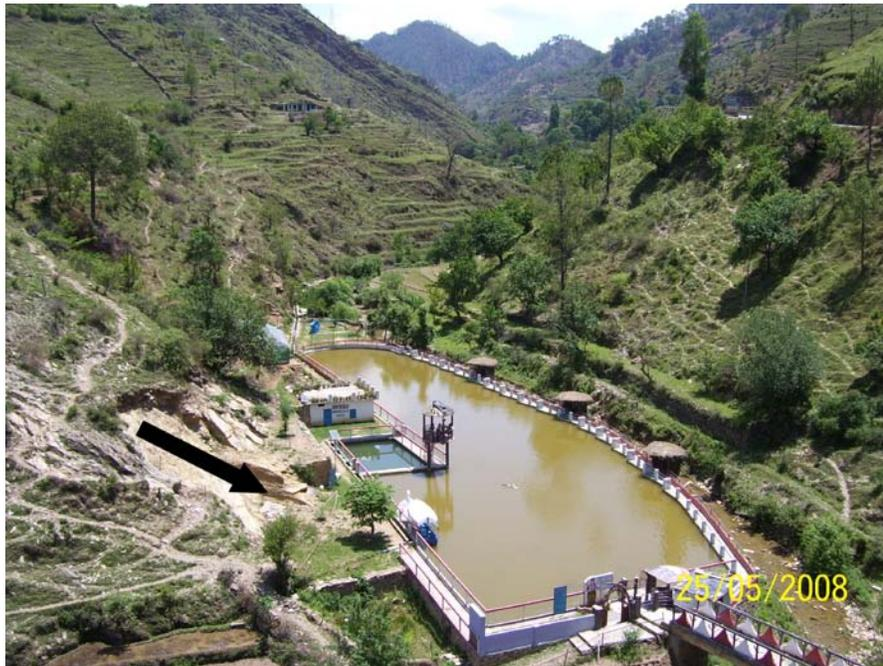
Fig.1. Hill side failure along planar discontinuities
